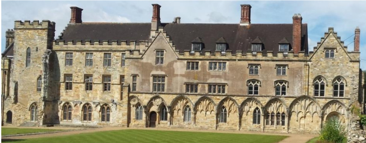
The west walls of the cloister can be clearly seen forming the lower part of the east wall of the post-dissolution manor house at Battle Abbey. Photo: © K Foord
